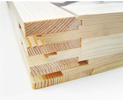
Shorted tenons allow stormproofing of sashes without breakout.
